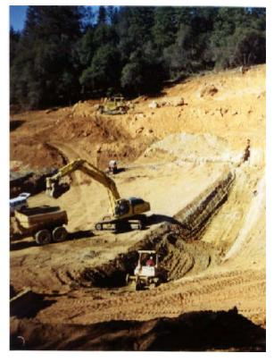
We provided recommendations and construction quality assurance for placement of 800,000 cubic yards of soil associated with the golf course. In addition, we provided recommendations for bridge construction, pavement design, and lime treatment of subgrade soil to facilitate wet weather construction.
