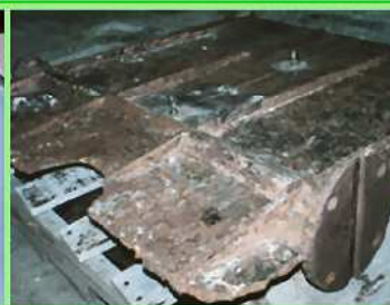
Severe rudder erosion caused by electrolysis and cavitation
