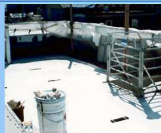
Aluminum, steel, concrete and wood decks can be coated as Duraflake has a 10-12% elongation property
