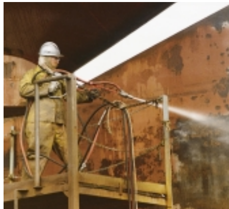
High Pressure Wet-Blasting System
