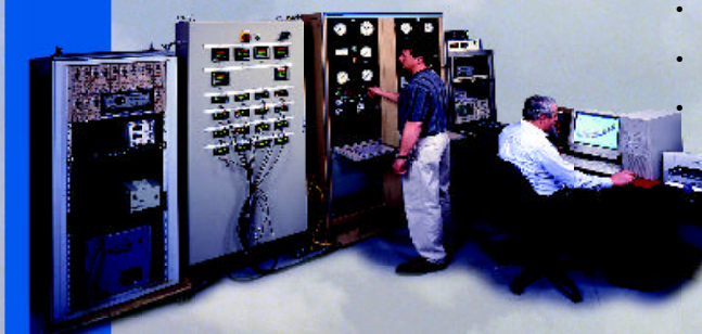
Spin Pit Control System and Data Acquisition Center
