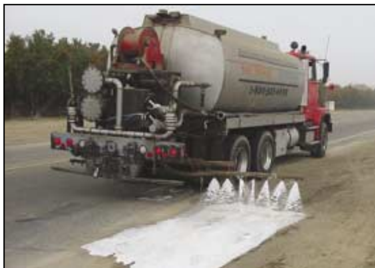
Soil-Sement® being applied.
