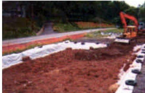
Bio-Pile Construction, Conesus Auto Service Facility
