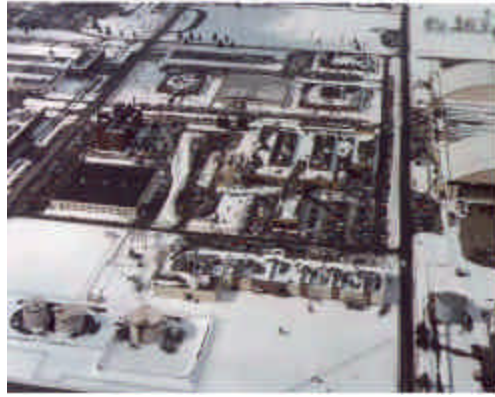
Rome Research Site, Aerial View
